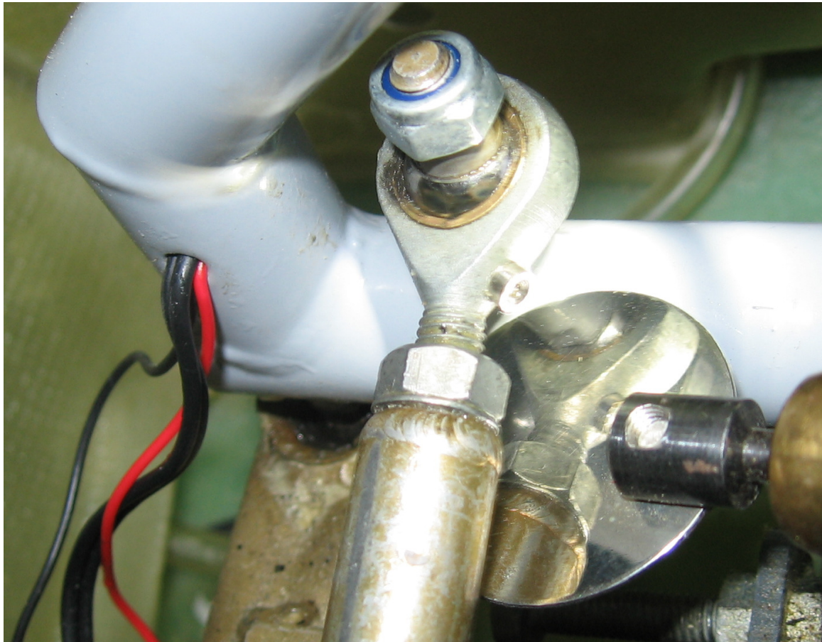
Inspection with a mirror, no X is existing, rod end must be replaced.
